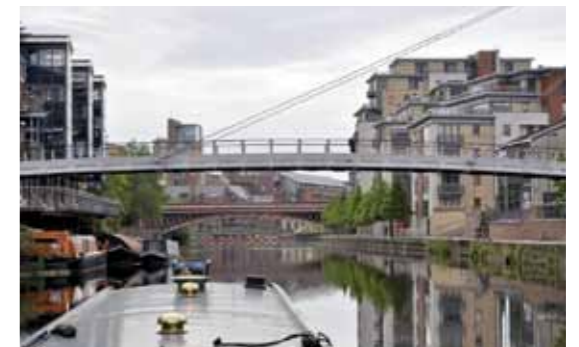
Aire & Calder Navigation, Leeds © Ray Hasmall
